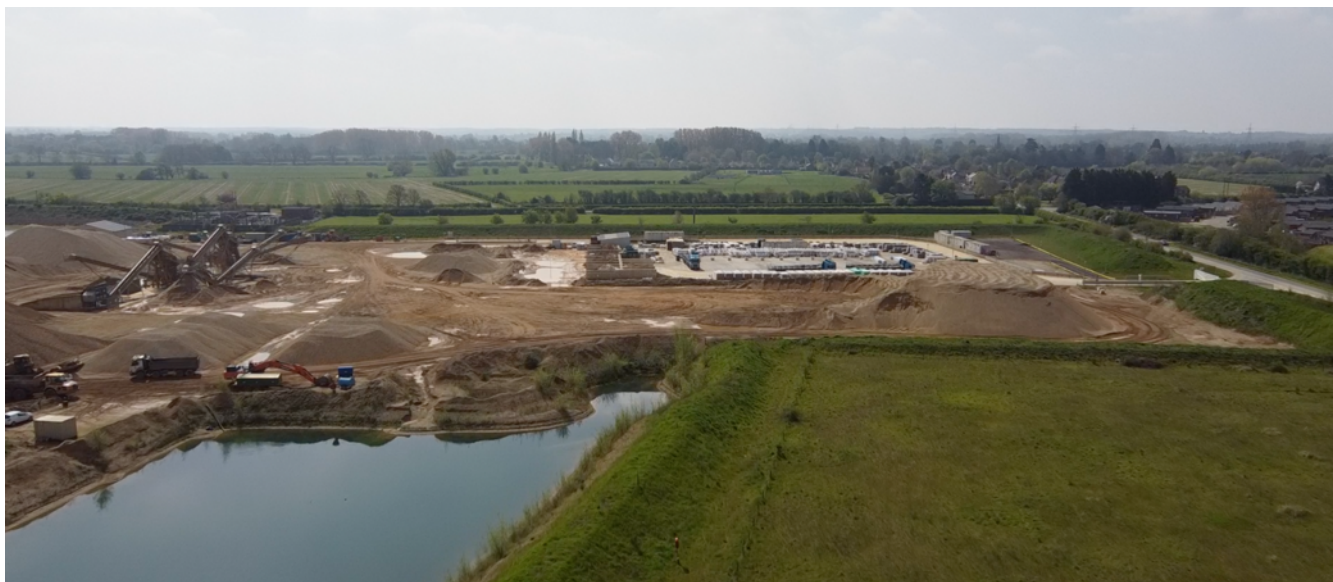
Fig 4: This is the Cemex processing and Bagging Plant – a similar scale industrial site is proposed in the top left striped field in this photo immediately in full view of the village.
